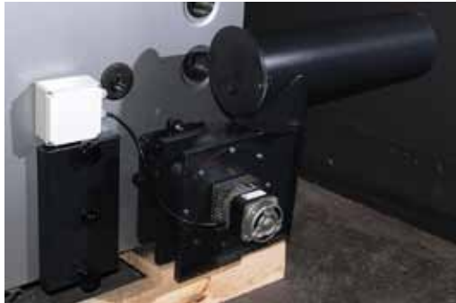
Extension duct installed on the blower. The product number of the extension duct is 5012981.
