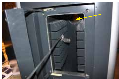
Open the convection cleanout hatch.
