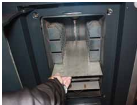
Remove all flue gas guide plates.
