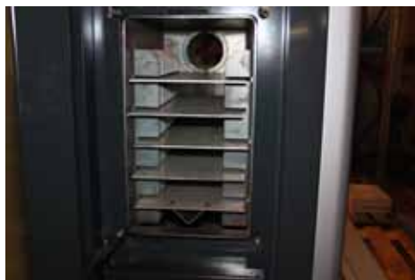
Remove all flue gas guide plates.
