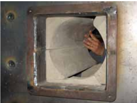
6. Upper part of front brick. The upper parts support each other with a suitably sized piece of wood in between, for example.
