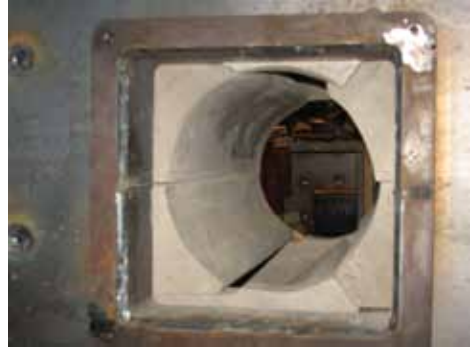
7. Upper parts of side brick (2 pcs) (pay attention to left- or right-handedness). Remove the temporary support then installation is complete.
