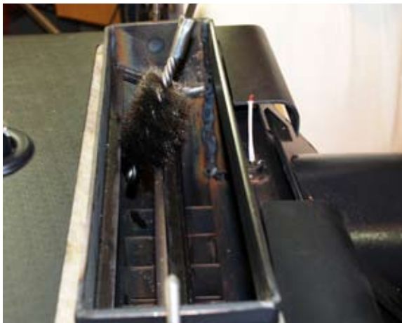
Cleaning brush is included in Ariterm pellet boiler delivery. Move the brush through the flues to sweep the ash from flue walls.
